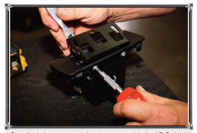
Once the holes were opened up to accommodate the HD Switch Panel mounting plate, both bolts were tightened up.
