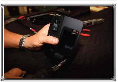
A little customization was required with the sPOD Universal Kit, but we had a Dremel tool and a steady hand. Remember to measure twice and cut once. Here, we're opening up the two holes to accommodate the mounting plate.
